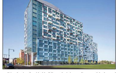
traditional ratio of an ideal building façade-to-square-footage. Moreover, the complexity of the cement panel color scheme strengthened the case for using a modular alternative, as did enhancements in project safety, logistics, quality control, budget and schedule
